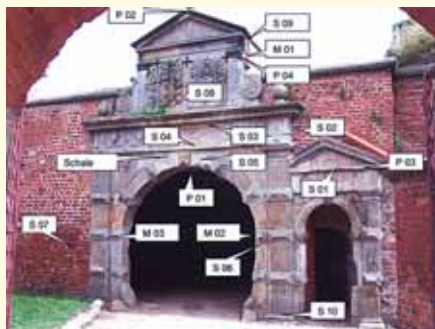
Mapping of the collected samples and their salt content (Documentation of a Restoration and Repair Project Sandstone Portal Dömitz)
